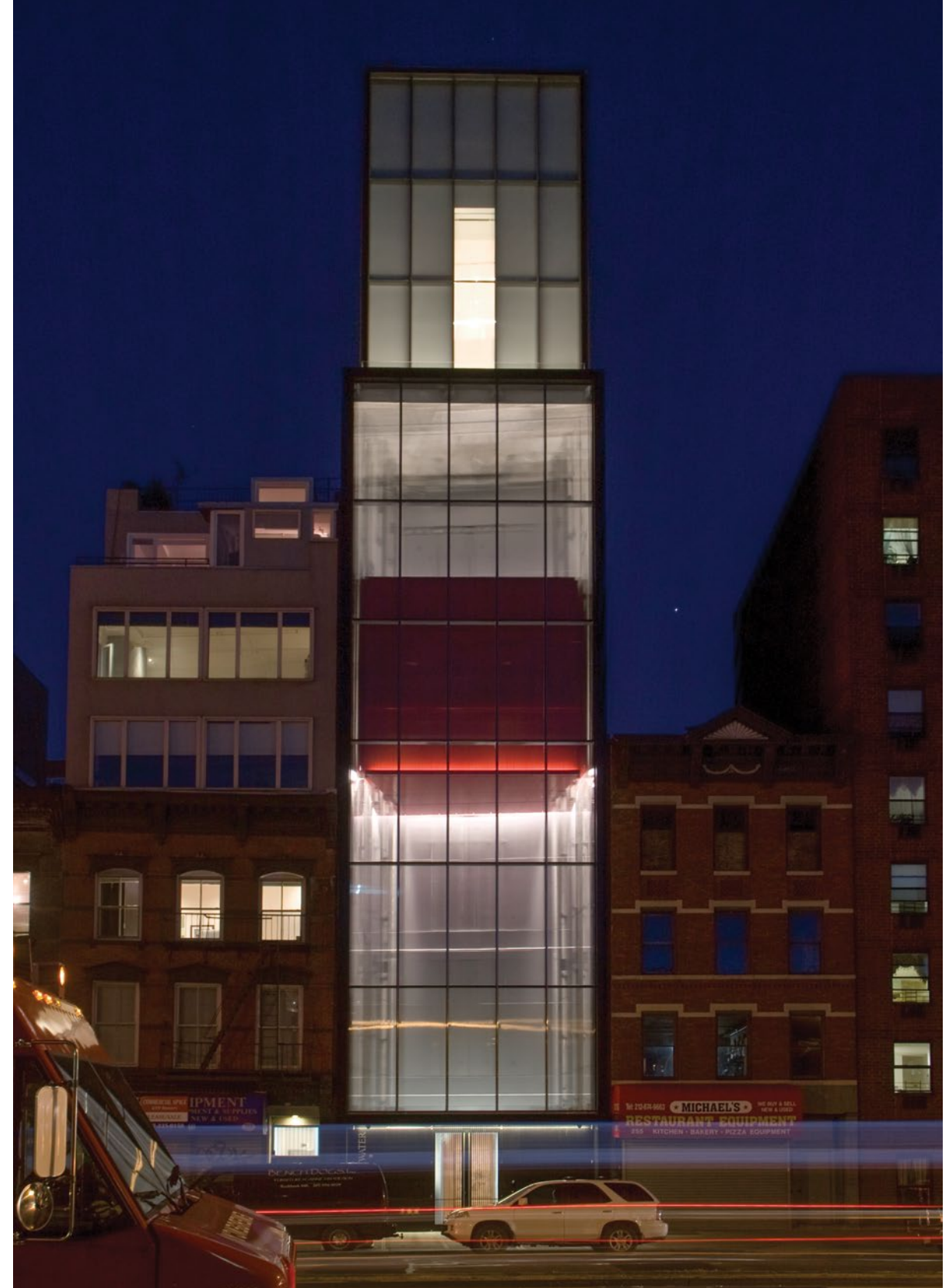
The red “moving room” at the Sperone Westwater Gallery in NYC includes embedded LEDs in its perimeter, roof, and around mechanical equipment to illuminate the full shaft no matter the position of the room. (PHOTO: Gabe Guilliams)
